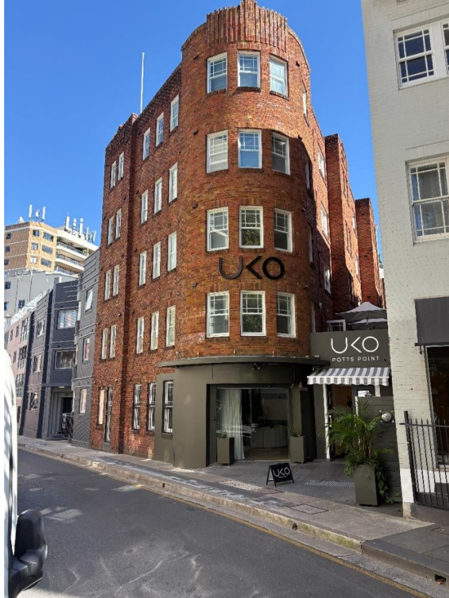
Figure 1: 15 Springfield Avenue, Potts Point, viewed from east
